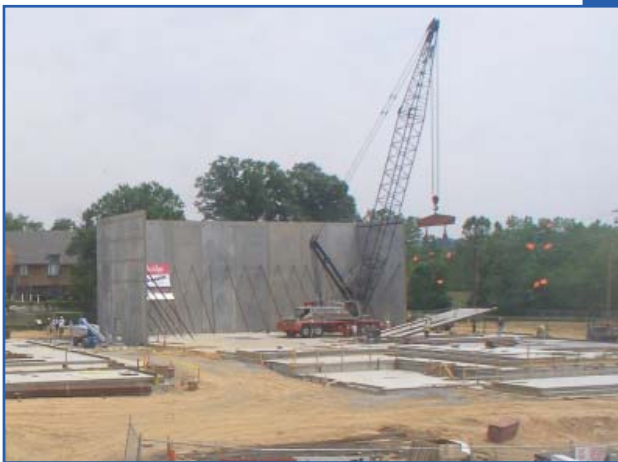
Erection of Warehouse tilt-panels.
