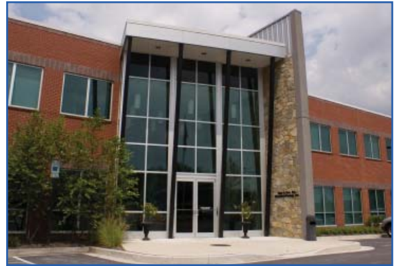
Multi-Story Office Building
